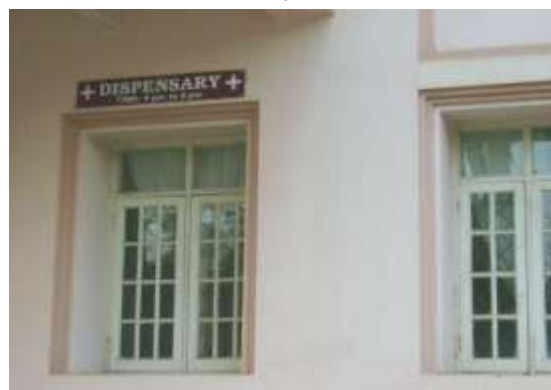
Dispensary in Hostels
