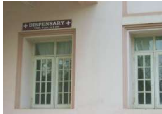
Dispensary in Hostels
